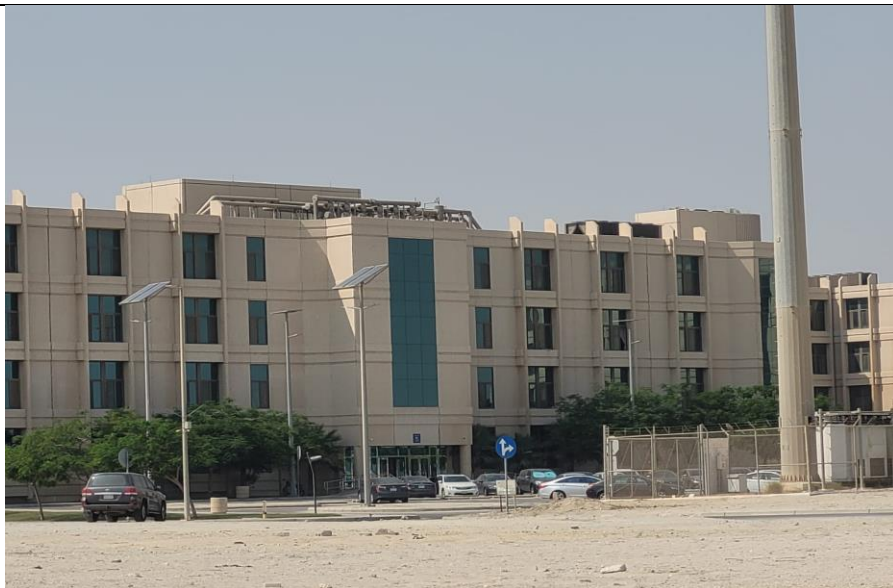
Solar Panels installed all over the campus to provide energy for the purposes of lighting, heating, cooling, running university laboratories, etc
