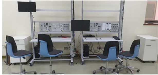
Power Systems Lab
