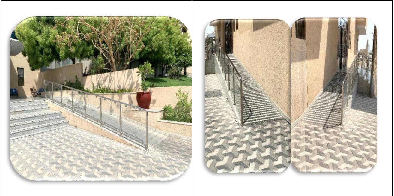
Ramp facility for Disabled at the entrance of every facility building of the IAU campus
