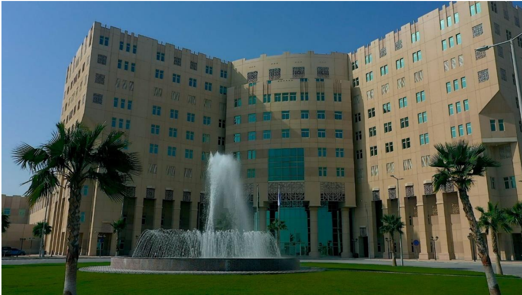
Treated water used in Water Fountains
