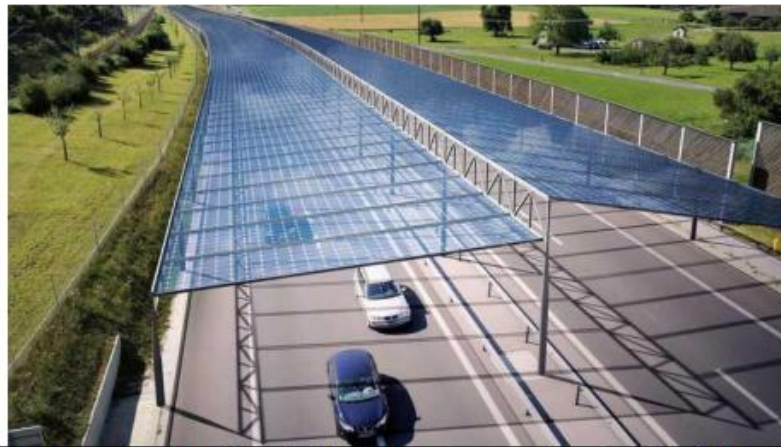
Photo solar systems installation initiative to reduce monthly electricity bill payments:
